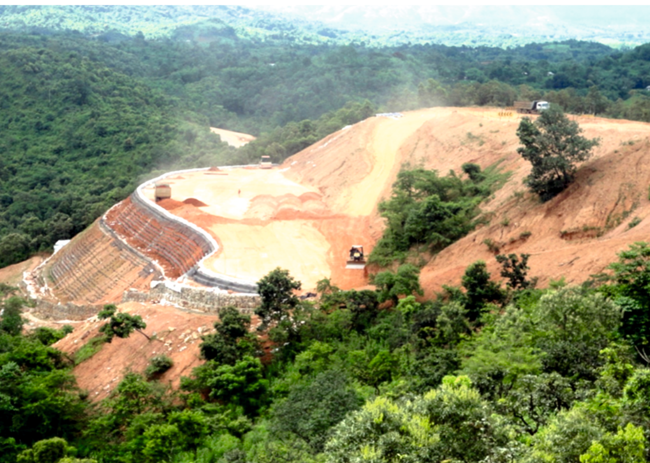
Stage 3: Reinforced soil slope - Completion of 18 Meter Height
