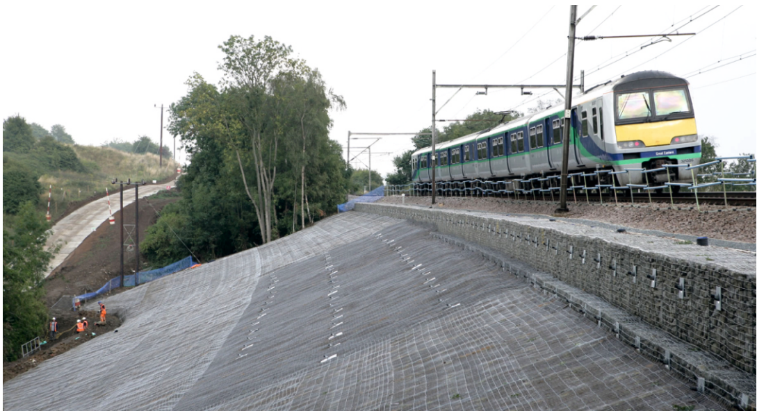
Rail Embankment using Geotextile
