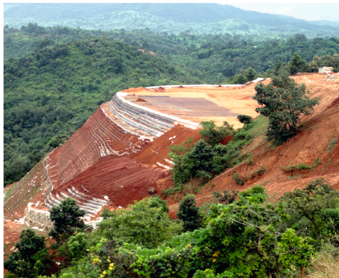
Stage 4: Reinforced soil slope - Completion of 27 Meter Height
