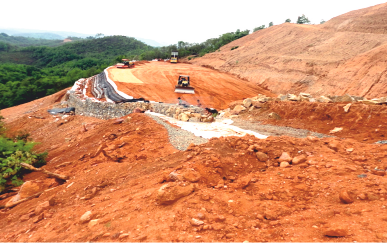
Stage 1: Construction of Gabion Toe.
