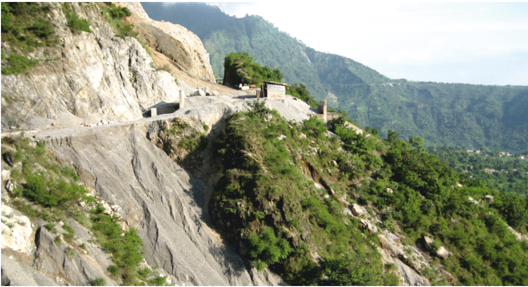
Reinforced Soil Slope for New Rail Line, Reasi (J&K), India
