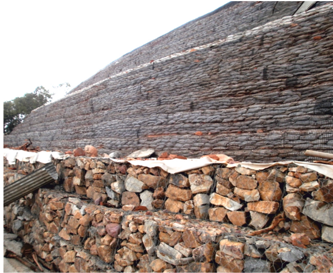
Stage 2: Reinforced soil slope - Completion of 10 Meter Height
