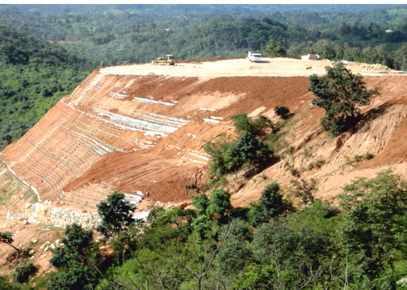
Stage 5: Reinforced soil slope - Completion of 43 Meter Height (2011)
