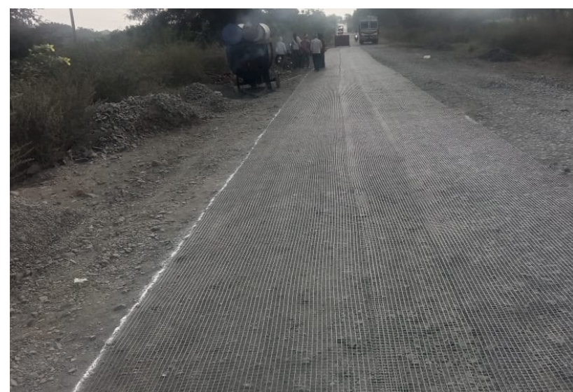
Asphaltic Reinforcement, Latur
